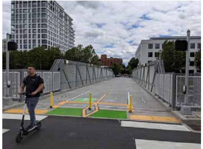
Figure 23. Path Delineation with on-path icons and symbols
