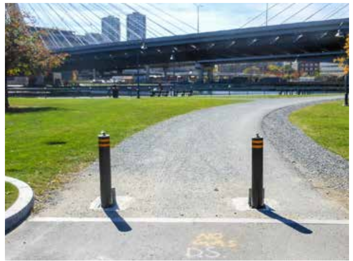
Figure 106. Retractable Bollards, Paul Revere Park, Boston MA
