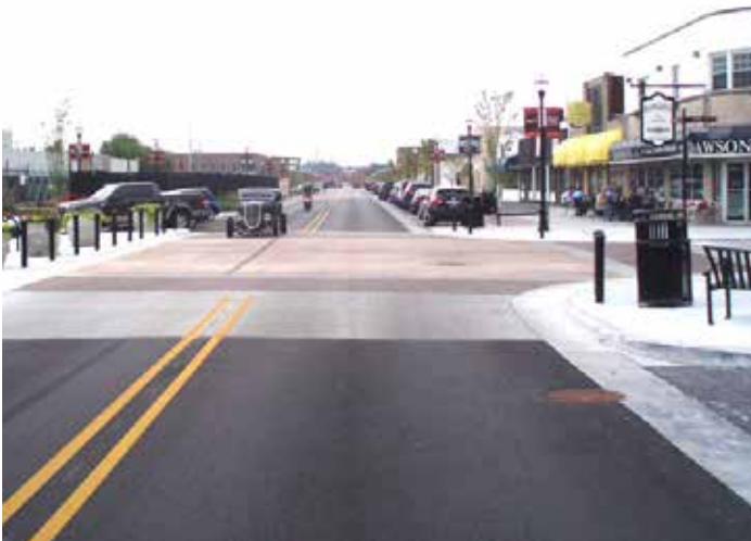
Figure 80. Raised Intersection - City of Oceanside, CA
