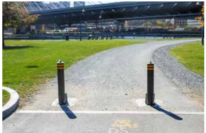
Figure 93. Retractable Bollards, Paul Revere Park, Boston, MA
