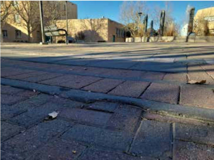
Figure 17. Uneven bricks on routes pose a danger to MMVs.
