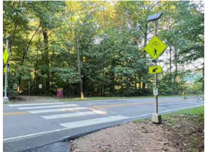
Figure 48. Rectangular Rapid Flashing Beacons in Raleigh, NC
