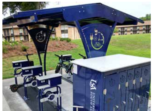
Figure 121. EnerFusion Inc Electric MMV Charging Shelter
