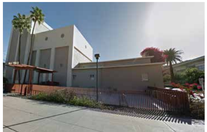
Figure 115. ASU Small MMV Valet Site (After)
