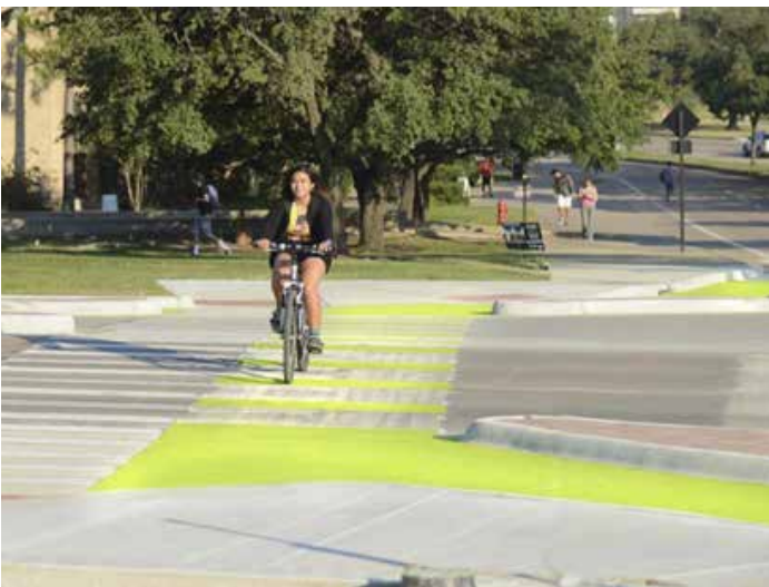
Figure 26. Texas A&M High Visibility Crosswalk
