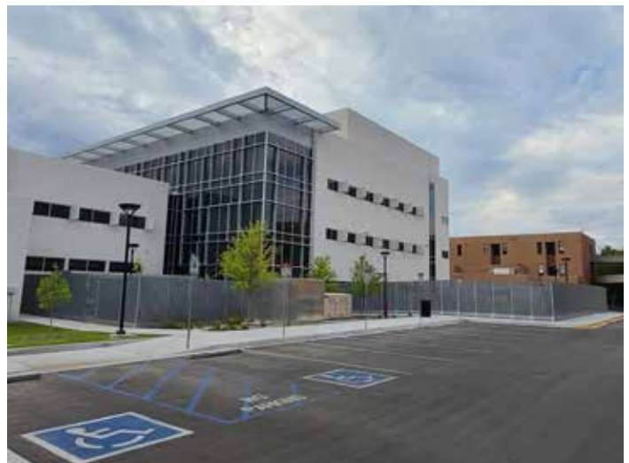
Figure 86. Existing Secure Bike Yard at PAIS
