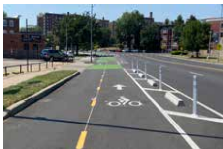
Figure 96. Roadway Cycle Track
