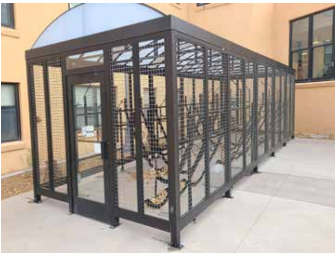
Figure 85. Existing Secure Bike Storage at Coronado Hall
