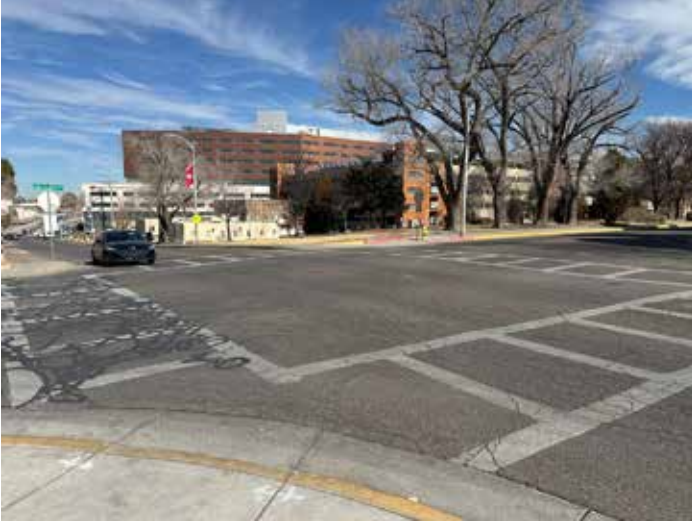
Figure 79. Existing Crossing - Yale and Las Lomas
