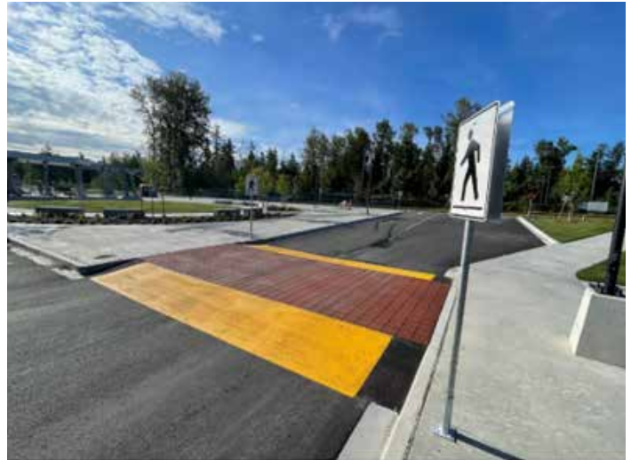
Figure 42. Best Practices Crosswalk Example - Raised Crosswalk
