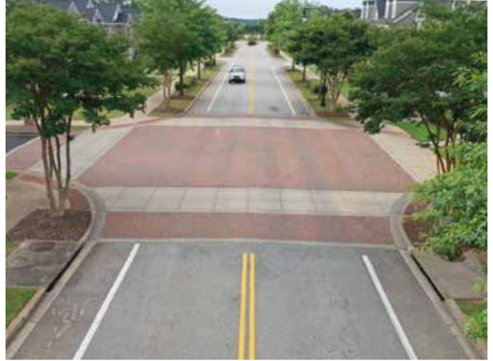
Figure 81. Precedent Raised Intersection Non-Signalized
