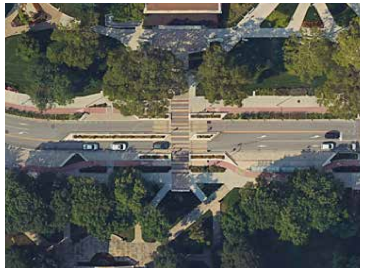
Figure 78. University of Pittsburgh Campus Perimeter Crossing
