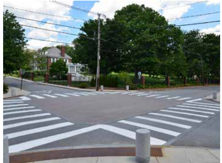
Figure 82. Precedent Raised Intersection, Tufts University
