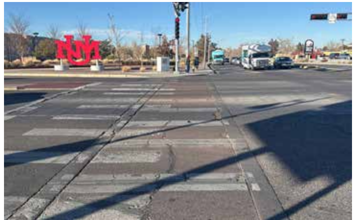
Figure 75. Existing Crossing - Girard and Central Ave
