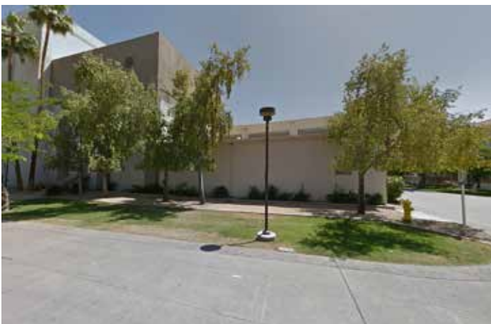
Figure 114. ASU Small MMV Valet Site (Before)
