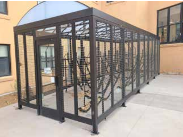
Figure 117. Secure Bike Storage at Coronado Hall
